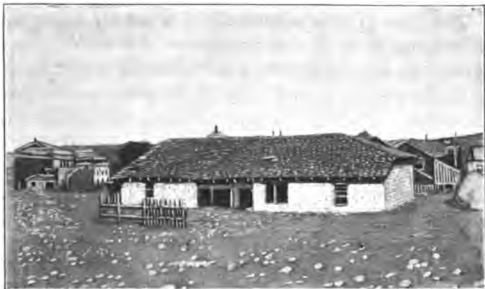
Old adobe house with modern roof
